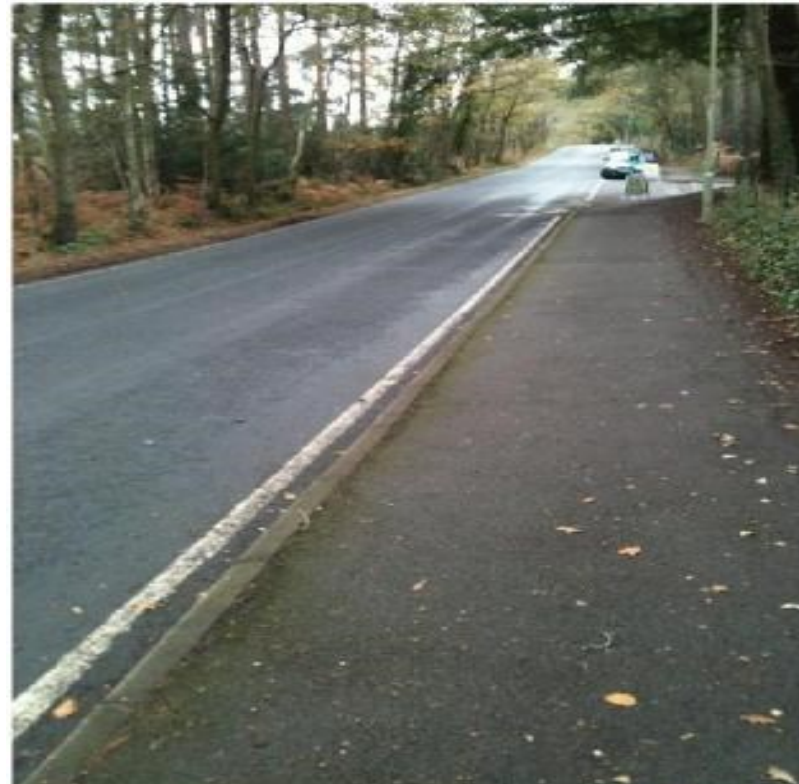
Figure 1. Drift Road looking west
