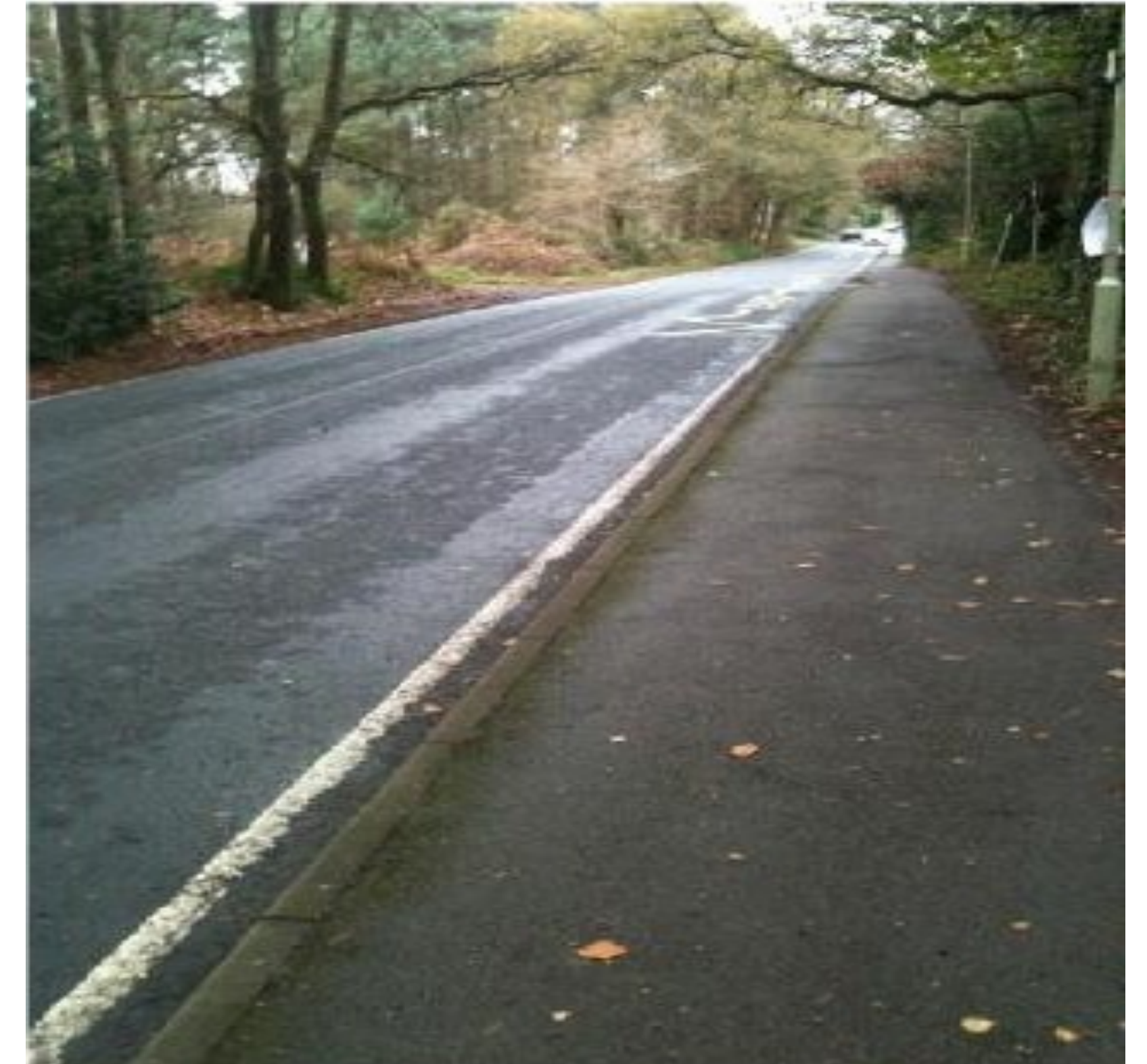
Figure 2. Drift Road looking east
